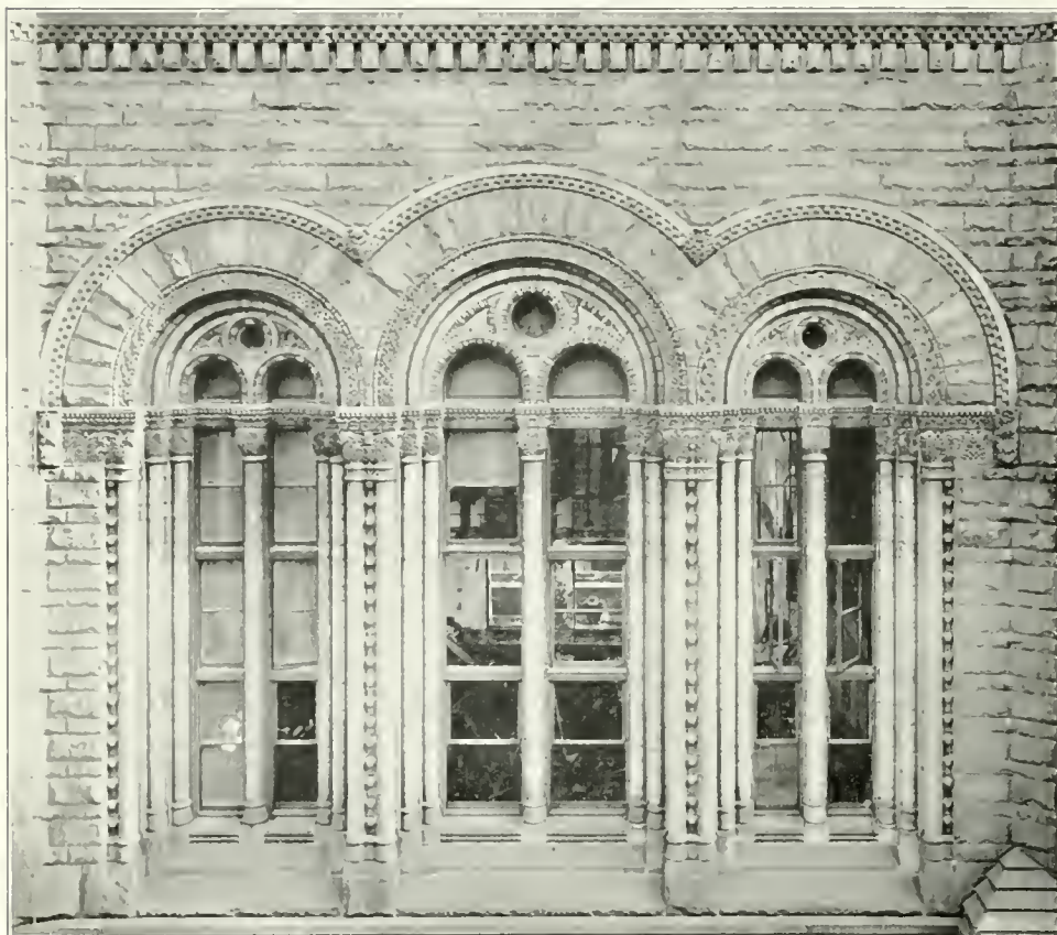
Fourth Street Window Arches, showing details of stone-carving. Photo. by Longley, 1911
